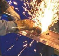
Type 18R plug used to grind I.D. bevels and flatten surface on rail frog section.
